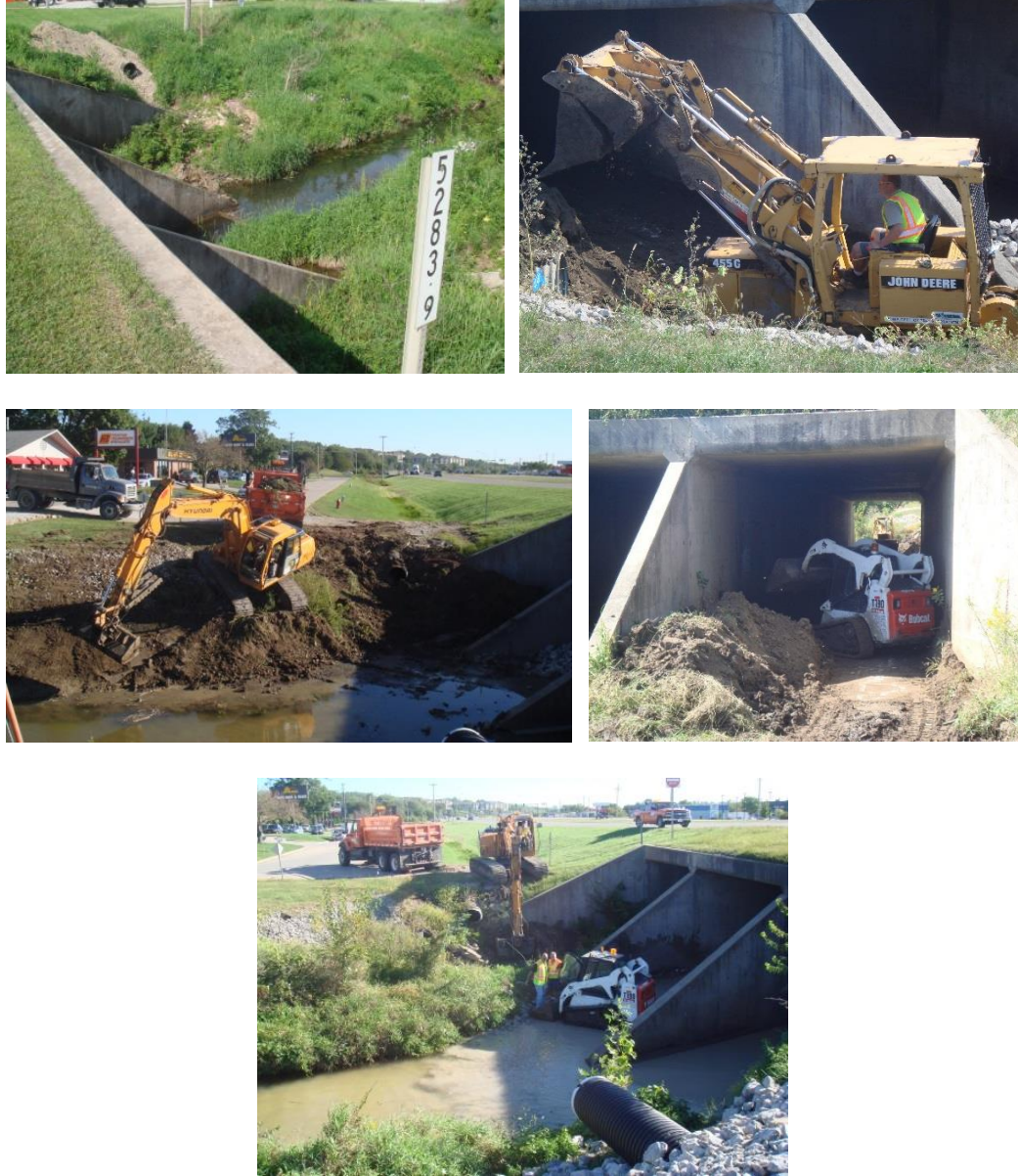
Figure 2.8 Culvert sediment cleaning involve excavator (Muste, 2014)
